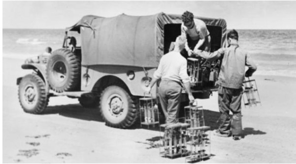
AWM image PO3332 015: December 1944, Mission Beach: Chemistry personnel loading Porton bubblers into a Dodge truck. The bubblers were used for measuring the concentration of gas.
