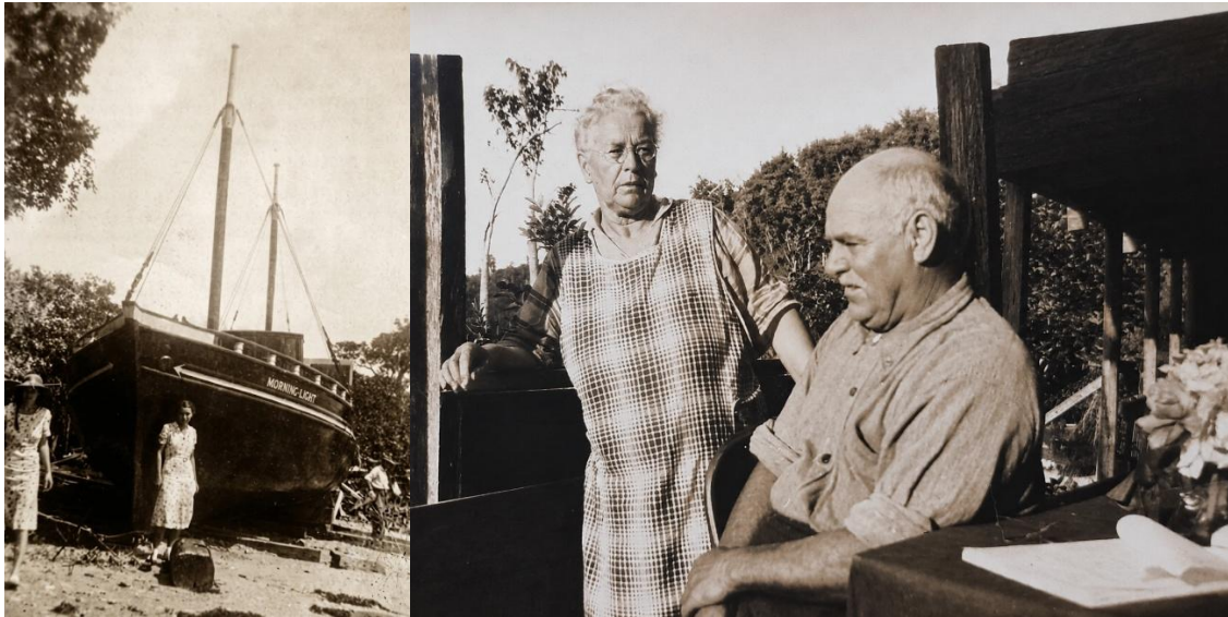
Left: Morning Light nearing completion. Image courtesy Kay Stephens.
