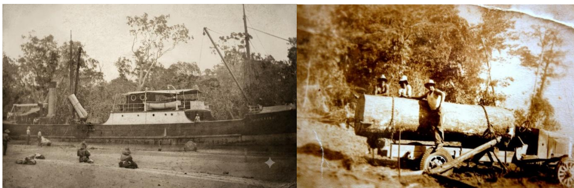
Left: Loading logs in Muff Creek. Right: Bert Wildsoet and Frank Garner continued the timber business. Images from Kay Stephens nee Wildsoet.
